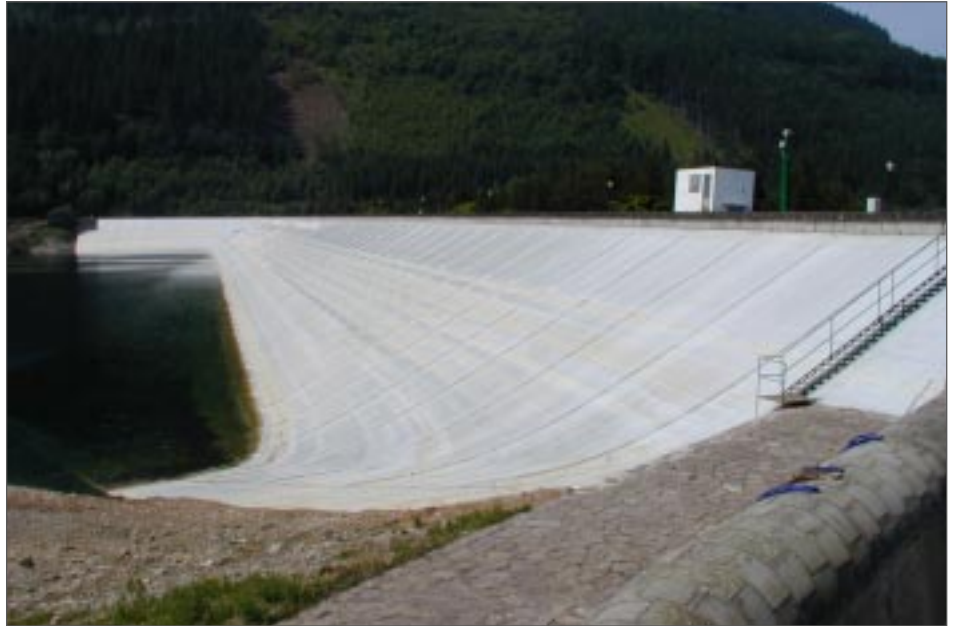
Reconstruction of the upstream face sealing (new geomembrane)
